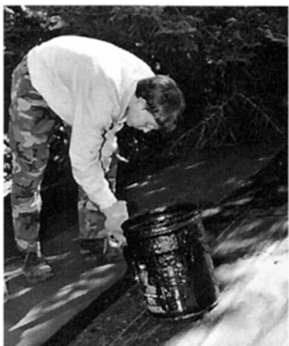
Bryan Dempsey leans over to brush more tar on the roof of Faul Cabin (00).
